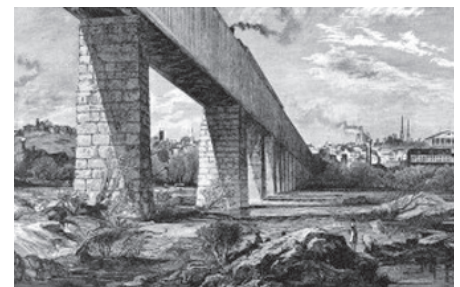
R&P Railroad Bridge (pre-civil war). Photo courtesy of the Virginia State Library.
