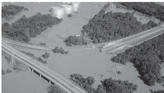
Flooding on I-95 in south Richmond prior to the construction of the floodwall.
